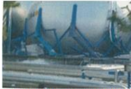
Figure 42 : Fractured support braces collapsed by strength ground motion
