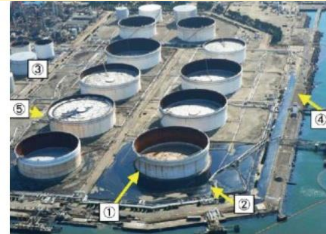
Oil leakage due to collapse of pipelines (Sendai JX Nippon Oil refinery)
